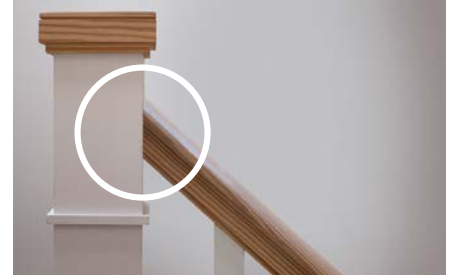
For use with angled railbolt for post-to-post at top of stairs
